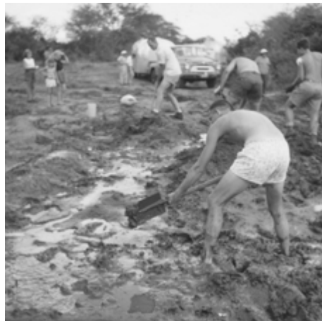
Rebuilding the Muddy Road
