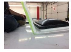
Once the surface has been cleaned, I like to use masking tape to form a bead line for the new sealant to be applied. This should be placed at the outer most area you want the edge of the sealant to be placed. Then apply the sealant to the perimeter of the fan and smooth the sealant with a putty knife. The sealant we use on the roofs currently is Adseal white part number 365330-01. Then pull the tape and you will be left with nice straight edges of sealant around the fan.
