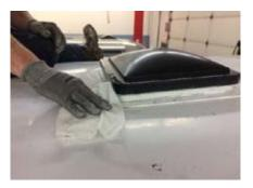
As you can see from the pictures above, a plastic style scraper is best to use as it has less chance of scratching or gouging your painted roof surface. After you have all the old sealant removed, you can follow that up with a good wiping with Denatured Alcohol so the new sealer can be applied to as clean a surface as possible.
