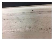
Here are a few photos of the sealer around a Fantastic Vent on the roof of the trailer. As you can see, it is starting to flake away and develop cracking in the sealant. This needs to be replaced.
