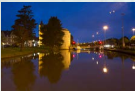
Kruispoort city gate at night
