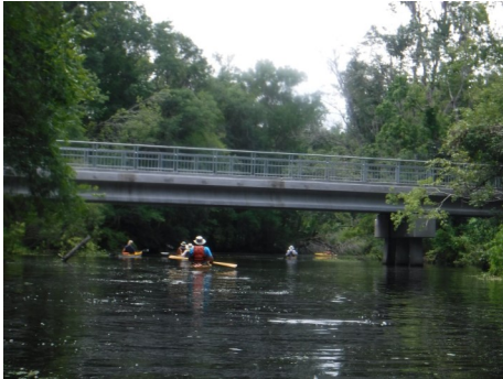
Deep Creek under Palatka-St. Aug. rails-to-trails bike path
