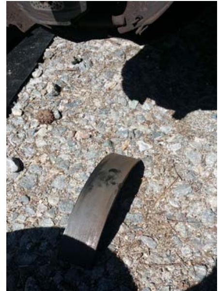
Lining material separated from the backing plate assembly (if this coach kept driving this material could cause a wheel lockup or failure of the brakes to operate).
