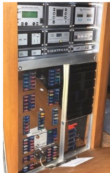
Most high tech control panel. 62 Globe Trotter.
