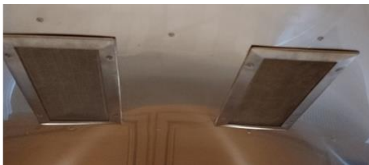
Return air grills (outside)
