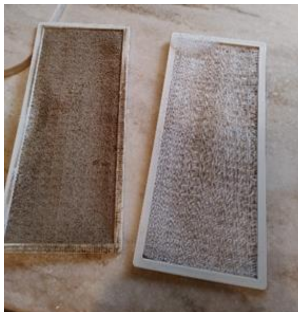
Inside screen filters: before and after cleaning
