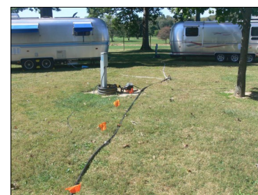
Water lines ready for use
