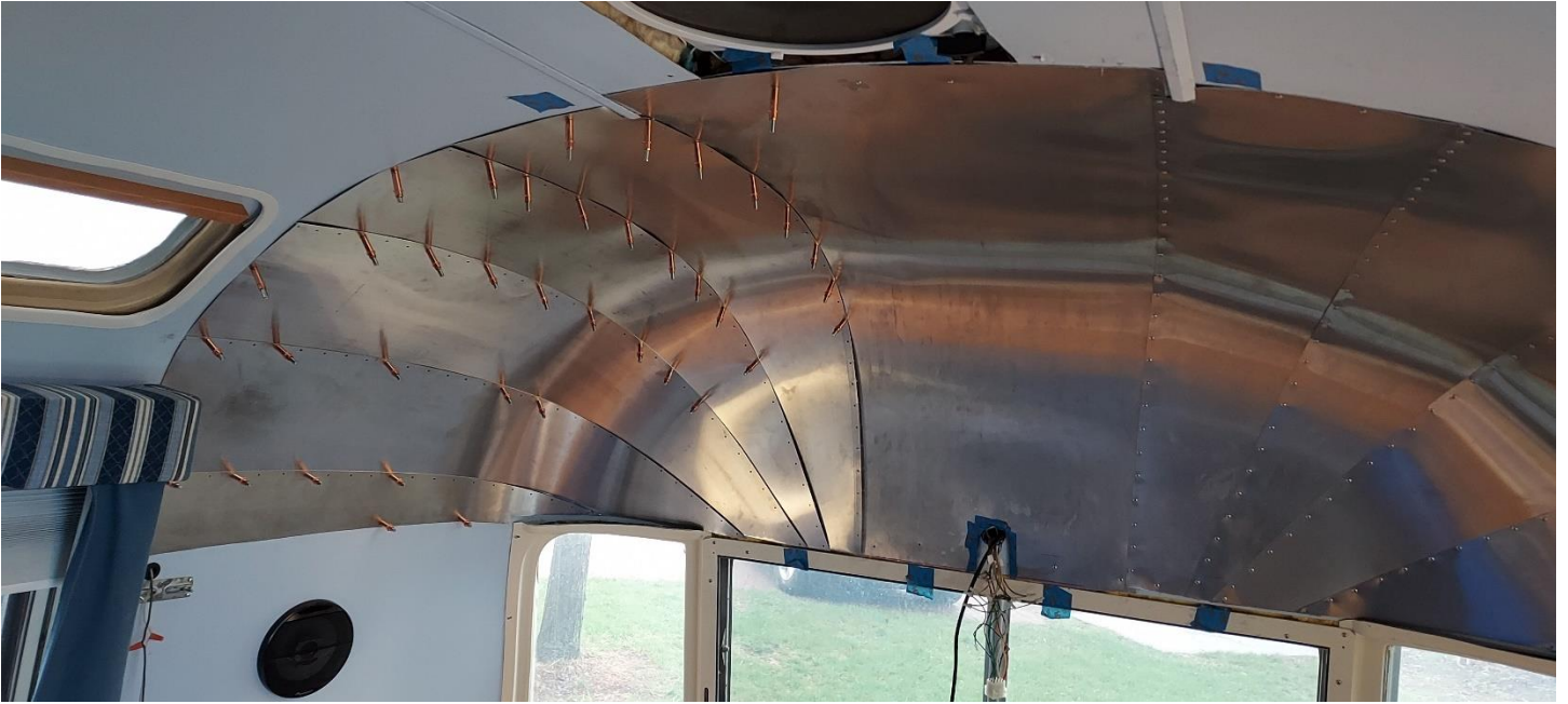
Port side all cleco'ed in place.
