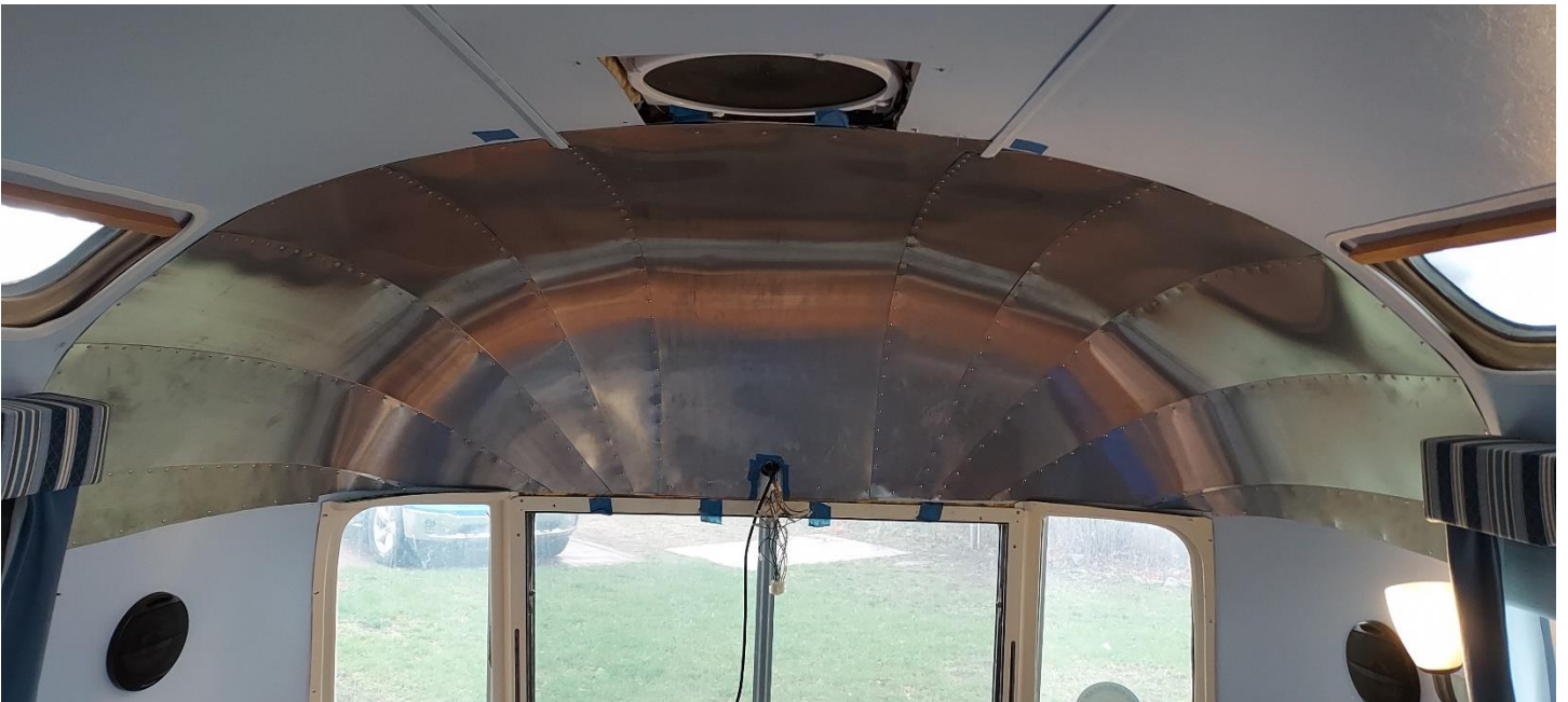
All 11 segments riveted in place. The two bottom segments on each side have about 5 inches cut off the bottom (basically split in half lengthwise) as I didn't need them to extend down the walls any further.
