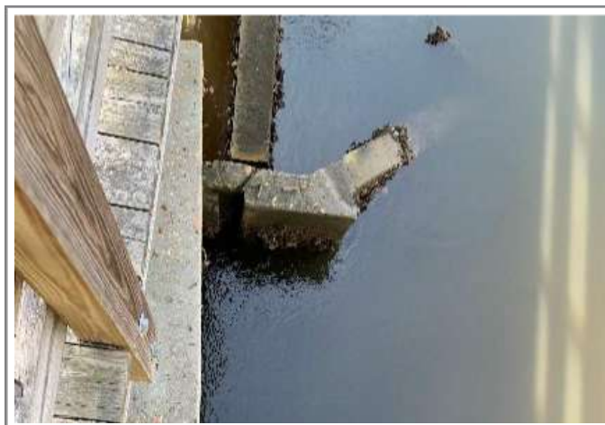
Below: Box Culvert below Bridge on Long Creek Trail
