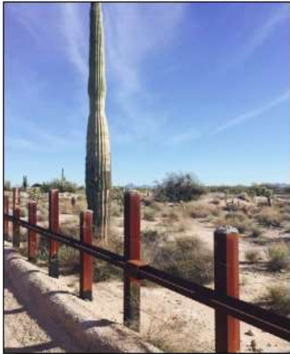
Organ Pipe Cactus Park's Arizona border with Mexico is only designed to prevent vehicles driving through!
