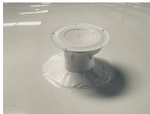
The Lippert 360 tank vent after installation.
