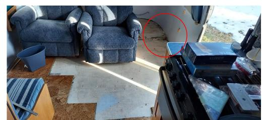
the damage that was in the middle of the floor came from the wall area in front of the window (circled in red).
