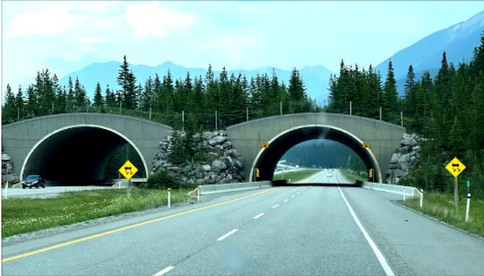
Wildlife overpasses between Banff and Jasper allow large animals to cross the highway safely.
