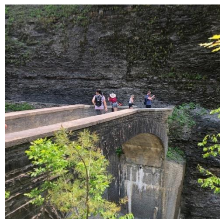
Footbridge linking the East and West side of the parks.
