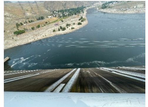
View from top of spillway looking down
