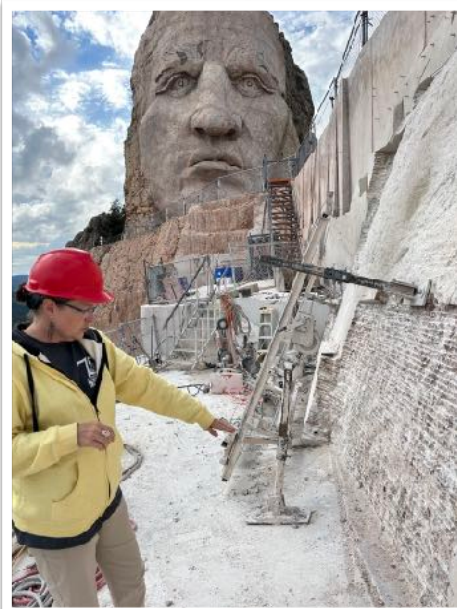
Gwen explaining the blasting process
