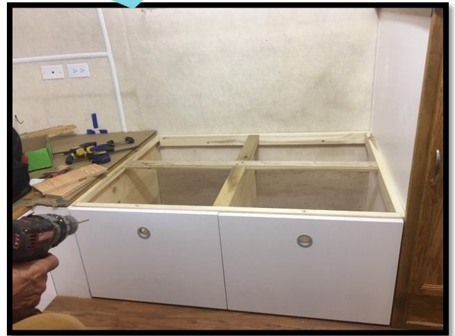
Completed doors under one side-with plastic rings that are part of wire management grommets for trim on finger holes in each door.
