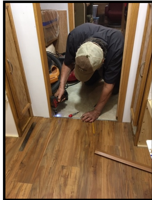
New flooring (Pergo-type) partly done & John putting down threshold trim between bedroom and mid-bath.
