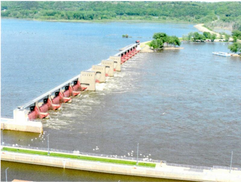
Lock & Dam 11 at Dubuque.
