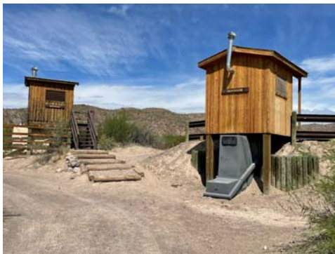
Check out these above ground vault toilets at the state campground. NO smell or flies at all.
