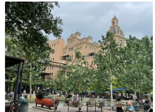
The Pearl District with the former Pearl Brewery at rear - now the very swanky Hotel Emma after a 20 year-long remodel
