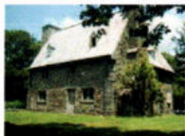
The Stone House in Guilford
