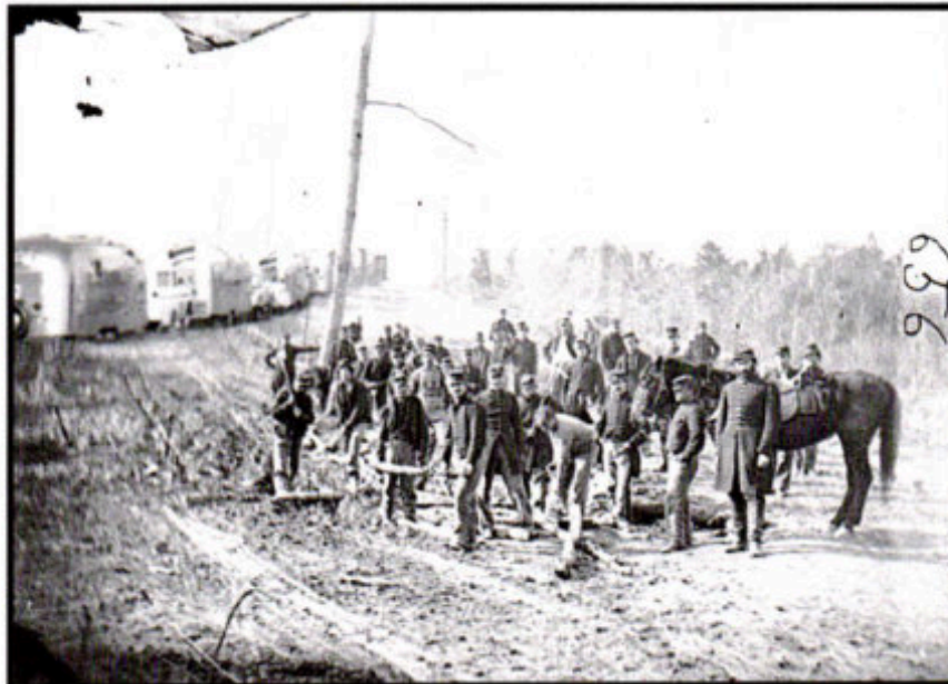
Engineers Building Corduroy Road Near Richmond, VA, June 1862 Recently discovered Civil War photo!
