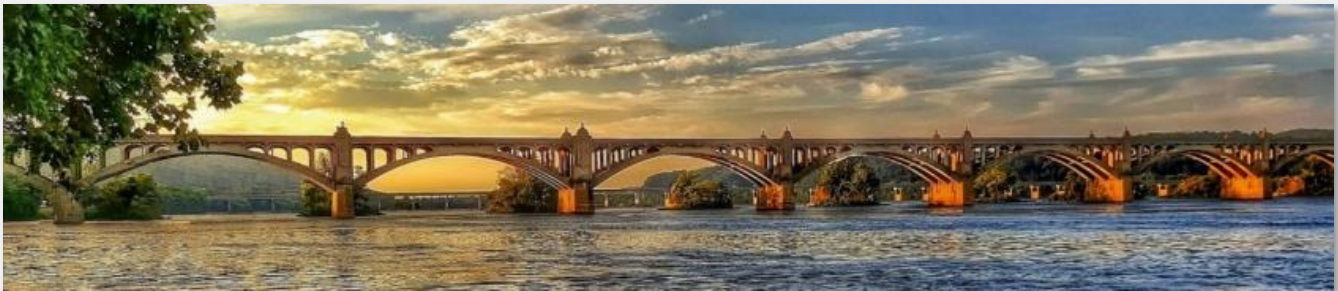
The Columbia-Wrightsville Bridge (also known as the Veterans Memorial Bridge or Route 462 Bridge) connects York and Lancaster Counties in Pennsylvania along Route 462 over the Susquehanna River. The bridge contains 48 spans, is 1.26 miles long, and is listed on the National Register of Historic Places.
