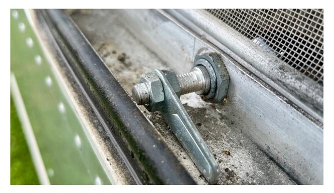
Then, go back inside and latch the window. The latch should now take a little pressure to pull the window in tight against the gasket. If the latch still turns easily without releasing it, go outside and repeat the nut tightening another full turn until the latch requires a little pressure to fold in the handle.
