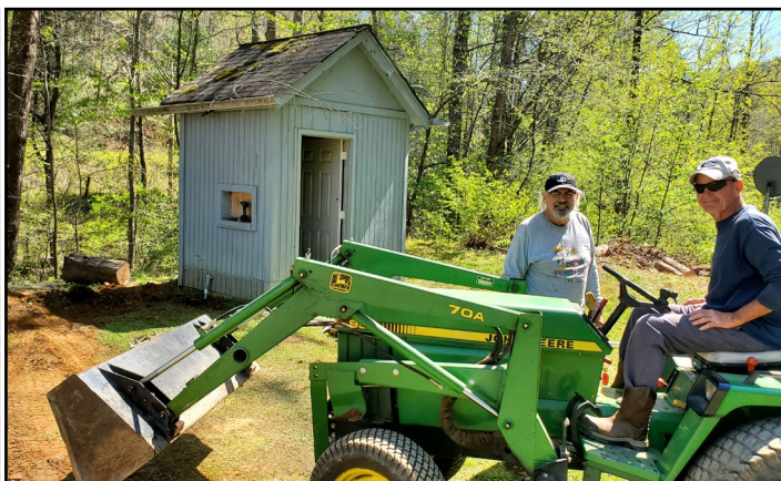
Mike Miller and Murphy Harrell after burying the underground power line.
