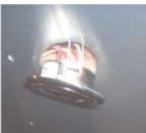
The halogen light is secured in the ceiling using two retaining springs. One spring located on each side of the light. These springs closely resemble a mousetrap. They are lifted upwards to clear the aluminum inside skin. Once the light is inside the ceiling the tension of the spring holds the light firmly into place.
