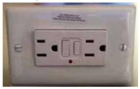
Purpose of GFCI: To prevent shock or electrocution. The GFI monitors current flow between the neutral and hot wires (it is not a fuse). If there is an imbalance in the flow of electricity it will trip the GFCI circuit.
