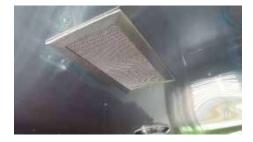
2. Remove the vent covers by pulling down out of the ceiling.
