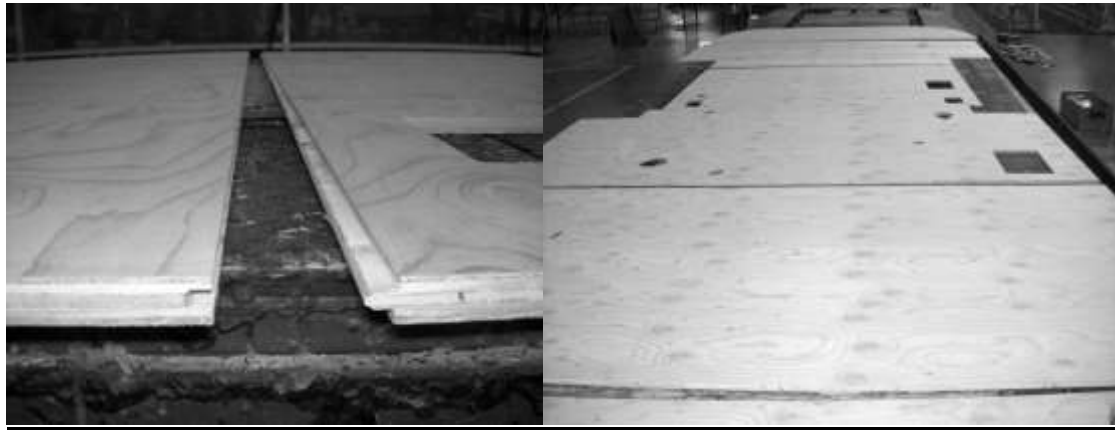
The flooring is 19/32" (5/8"), tongue and groove Exposure 1 Grade Plywood.
