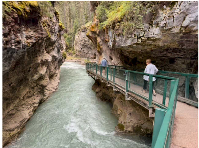
Cantilevered walkway in Johnston Canyon
