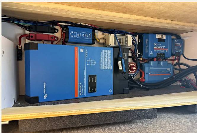
The MultiPlus and the distributor, before the lid went back on
